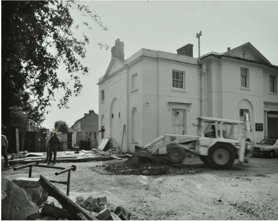
Commencement of extension works August 1981
