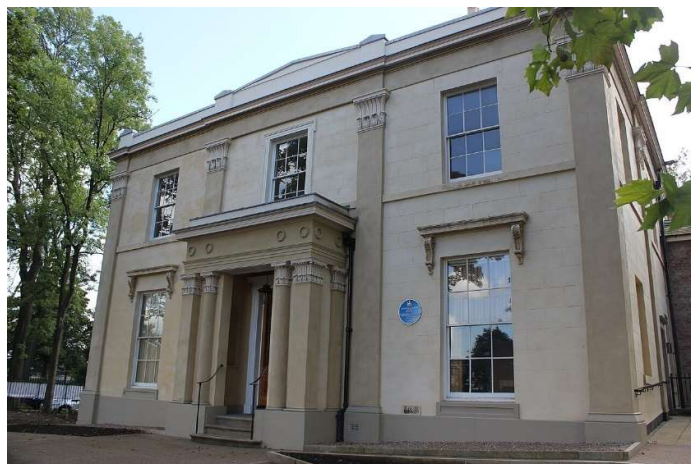
Elizabeth Gaskell's House Manchester following restoration works completed in 2014
